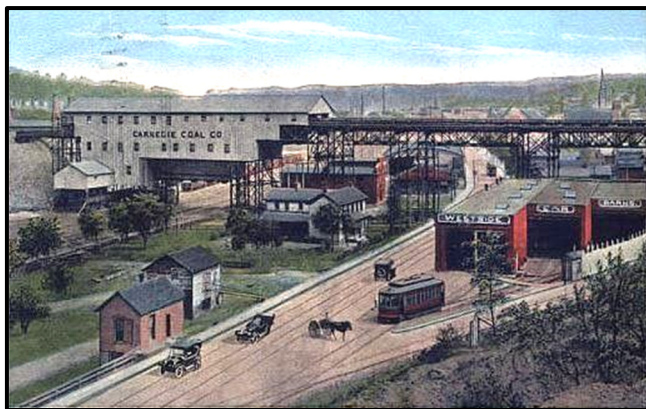
Top: Another view of downtown Charleroi, Pennsylvania, from an old postcard. Above: Streetcar barns and the Carnegie Coal Company in Charleroi. Right: The First National Bank in Charleroi. Many recently constructed buildings were present when the Jan Kopach family settled here after 1910.
