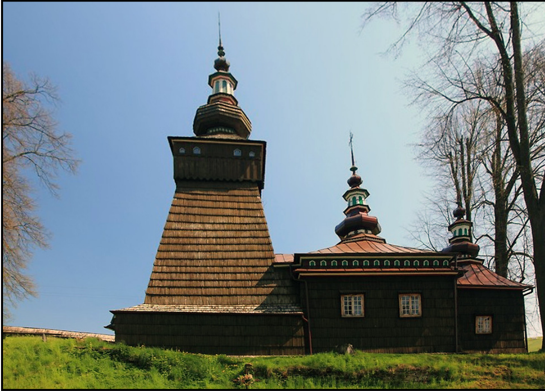
Above: Former Greek Catholic Church of Dormition of the Mother of God in Andrzejowka, Poland, that was built in 1864. Today it operates as a Roman Catholic Church. It replaced a much older building, which had a bell made in 1484.
