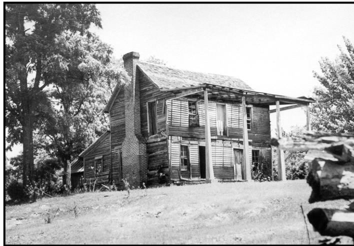
Above: Home of Wiley and Lucy Capps Crowley (4 th Great-Grandaunt) built about 1840. The home was the oldest residence in Greene County, Arkansas, before it was torn down in the 1970s. It was located across the highway from Warren's Chapel. Below: Crowley's Ridge State Park. Crowley's Ridge was named for Wiley's father, Benjamin Crowley (1758-1842).
